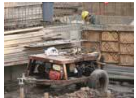
Ironmaster at work in the toughest environments of Ground Zero, NYC
