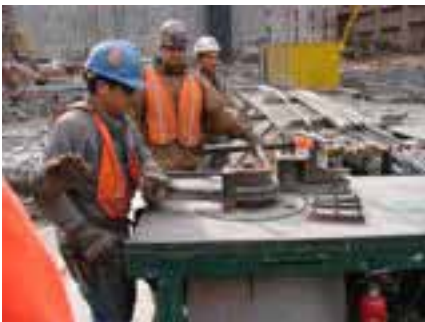
NYC Ironworkers bending rebar at Ground Zero
